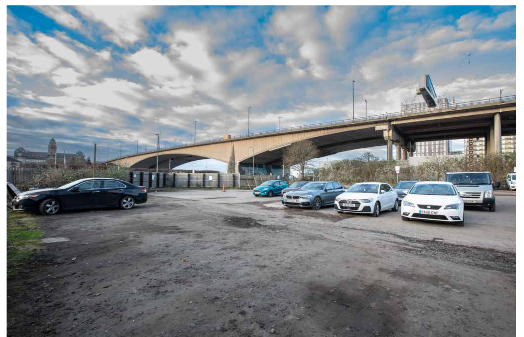
View from site to Kingston Bridge
